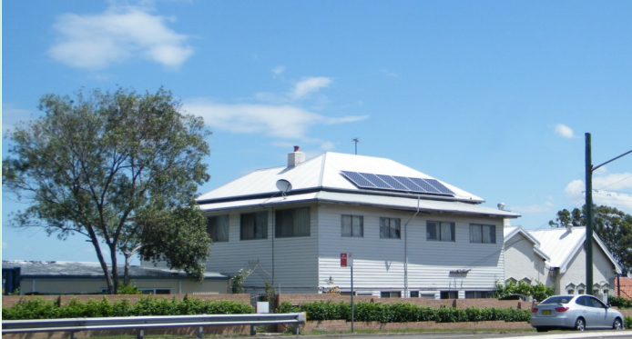
Sydney Centre Main building views from North East
